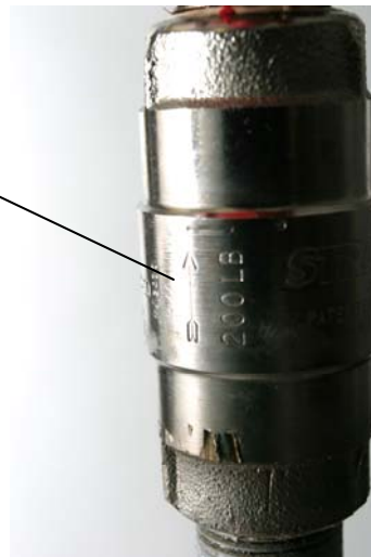
Fig 2: Check valve close-up. Note: Flow-indicator arrow. It must point up.
